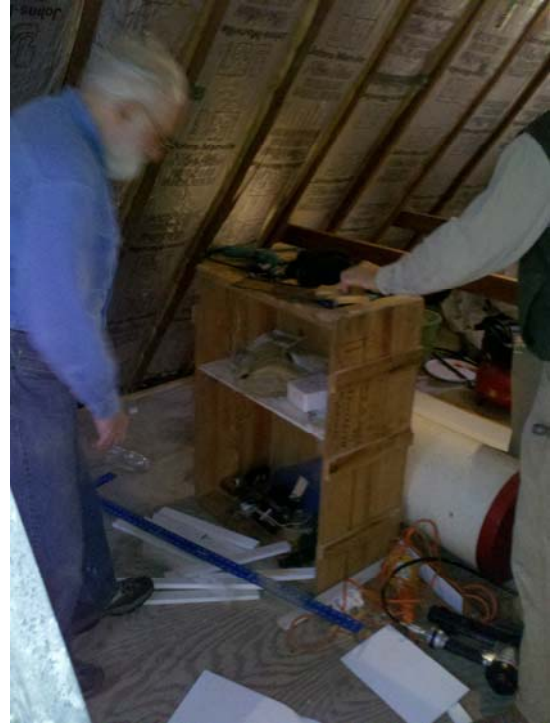
Jay Miller helped measure and cut the panels to size.
